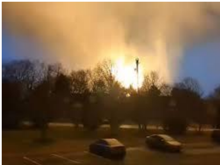
A large explosion was caused when the tornado hit an NES substation in Madison, TN. Image via: BrandonDavisBD/Twitter
