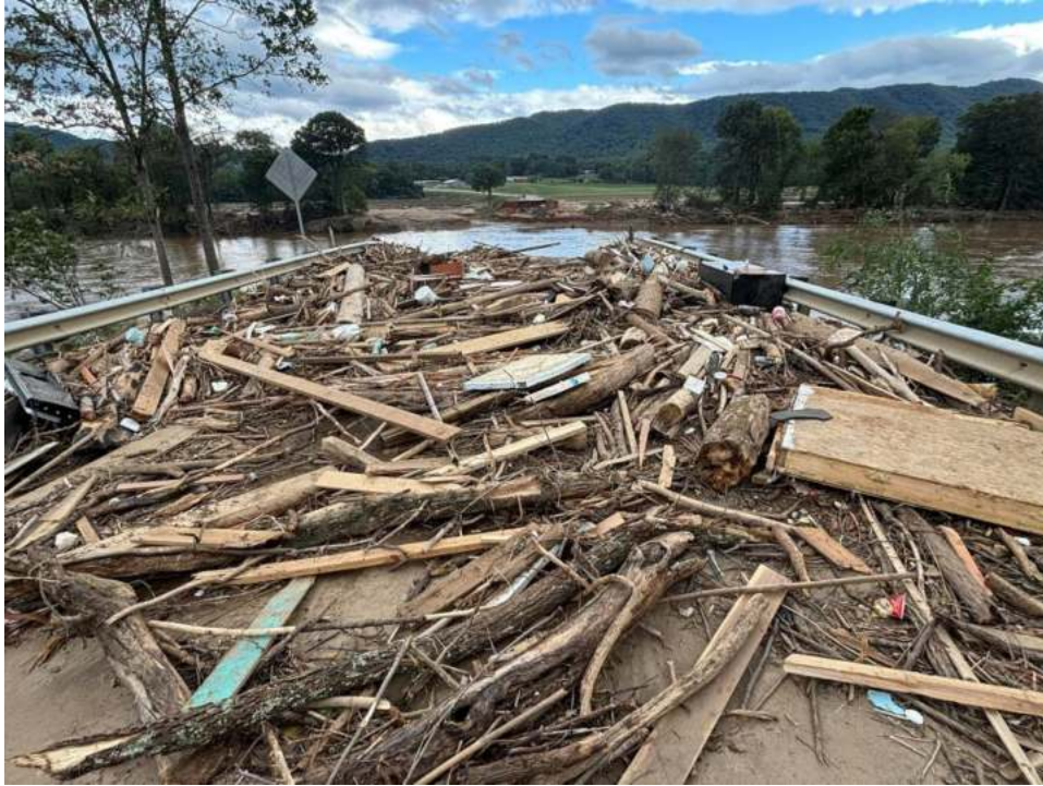
Debris near what was Taylors Bridge on State Route 81 in Washington County, TN Source: Facebook
