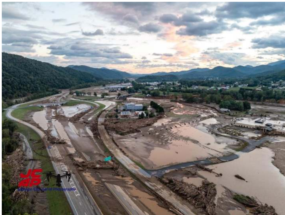
Area around the I-26 Jackson-Love Exit in Erwin, TN after the flood including the Unicoi County Hospital on the right side of the image. Source: Johnson City Aerial Photography
