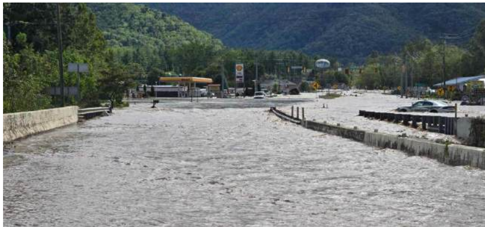
Doe River flooding on Hwy 19E in Hampton, TN. Source: Facebook, Elizabethton/Carter County Priority News & Alerts
